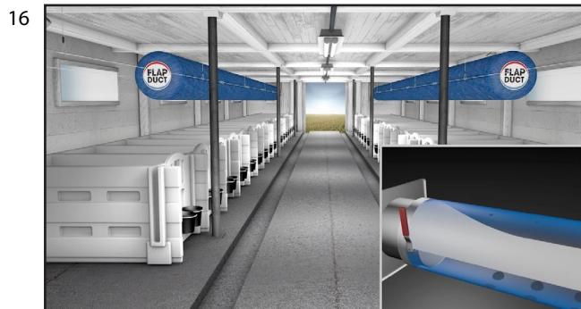
In warm weather, turn the variable speed fan to high, increasing air flow and position the internal membrane to the top of the duct using the lever control mechanism.
